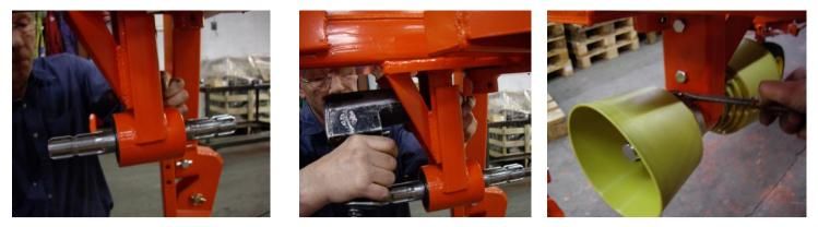
Step 10: Fit the position rod between the frames
